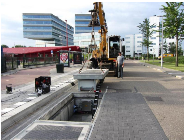
Caption: "Inductive Power Transfer" (IPT®) in use for electric buses: installation of a 60 kW charging module in use at a bus station with 120 kW power. In the future, IPT Technology GmbH will serve this segment directly.
